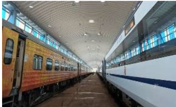
Vande Bharat Mumbai Central Pit Line Shed
