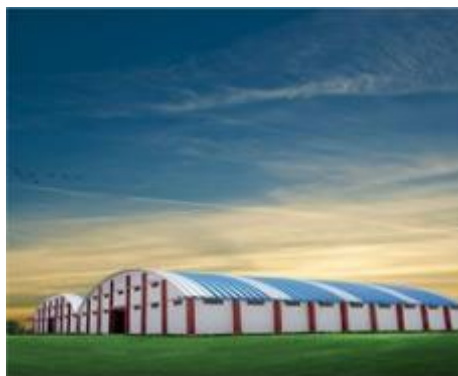
Roof with RCC Structure
