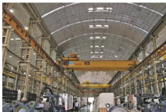
Roof with Overhead Crane
