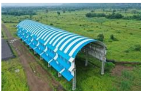
Roof with Steel Structure
