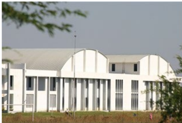
Roof with Semi/Half Arch
