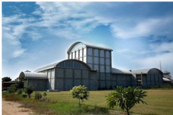
Roof with Differential Height
