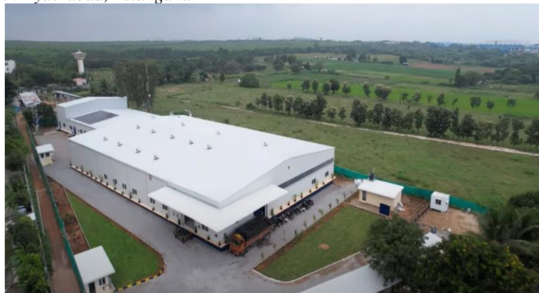
Vegetable processing facility, quality lab and biotech lab
