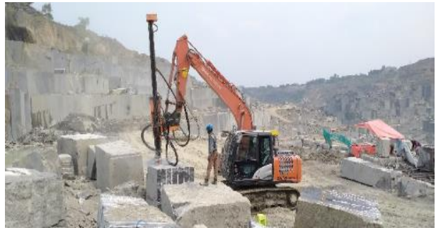
Excavator-mounted Mechanical Drill
