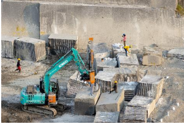
Excavator-mounted Mechanical Drill
