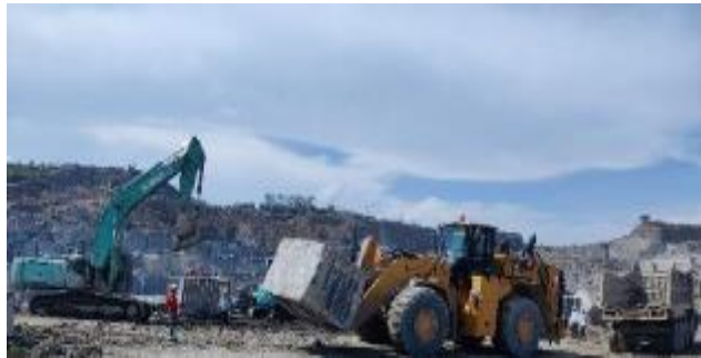
Wheel Loader with Excavator in foreground
