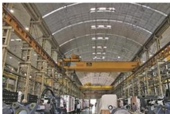
Roof with Overhead Crane
