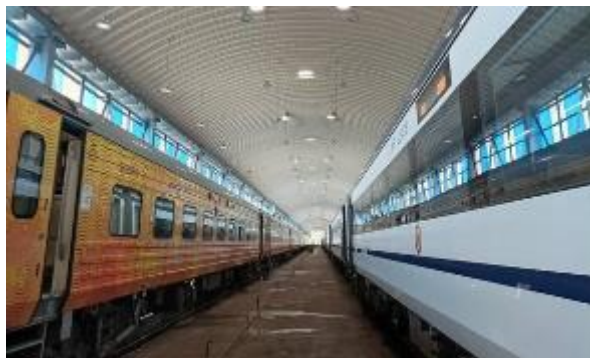
Vande Bharat Mumbai Central Pit Line Shed
