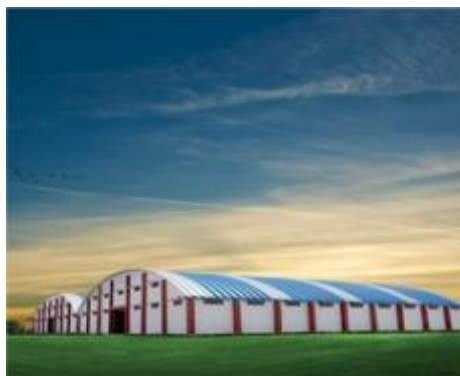
Roof with RCC Structure
