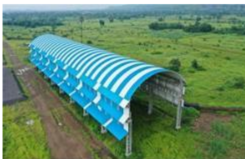
Roof with Steel Structure
