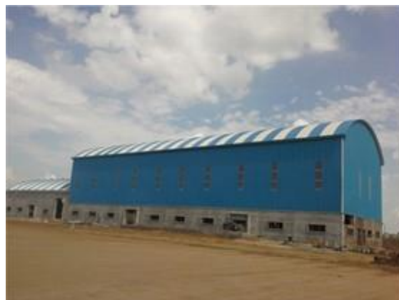
Roof on an Elevated Base
