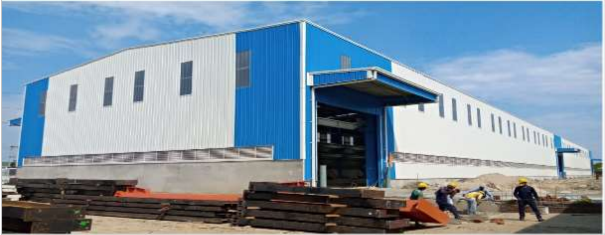
Tamil Nadu Manufacturing Facility I
